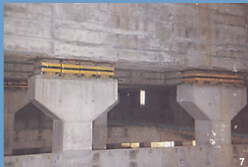
Fig. 1, 2 Recesses in the formwork above column heads
