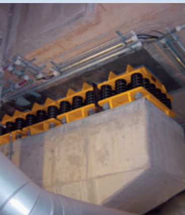
Turbine Column Head
