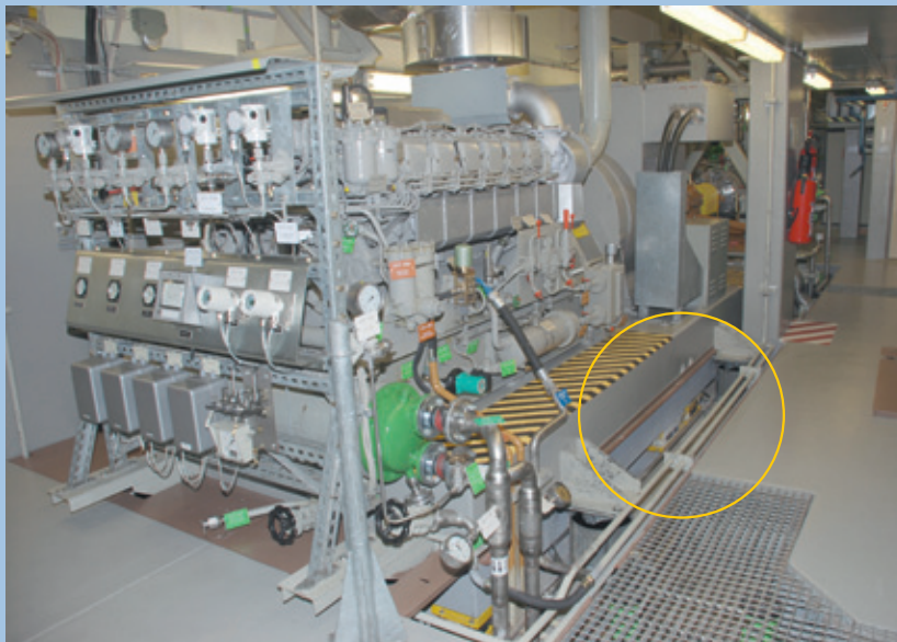
Spring Supported Emergency Gen Set (MTU)
