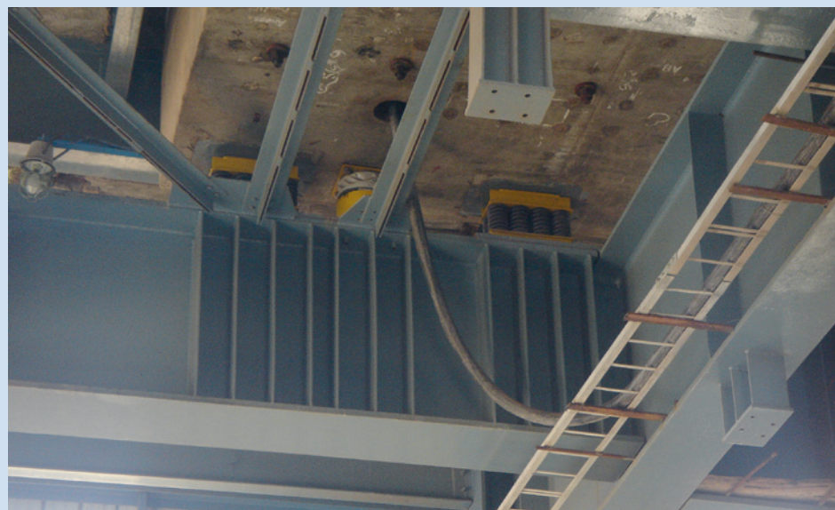
Ring Granulator on Steel Substructure
