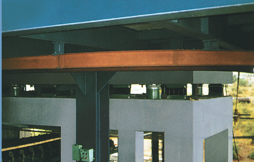
Ring granulator foundation with RCC substructure
