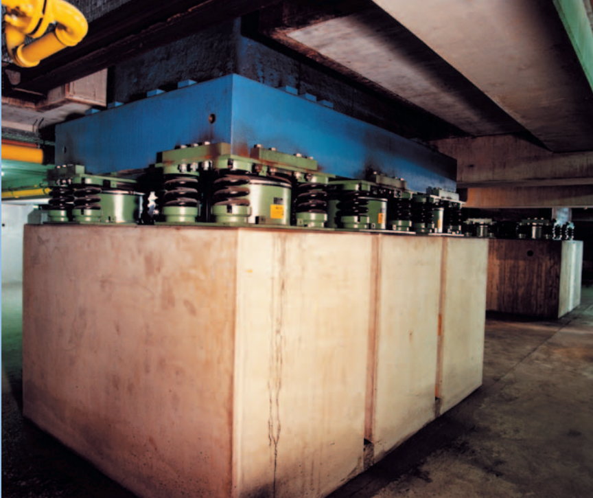
Spring Support of a Forging Hammer with Additional Steel Plate
