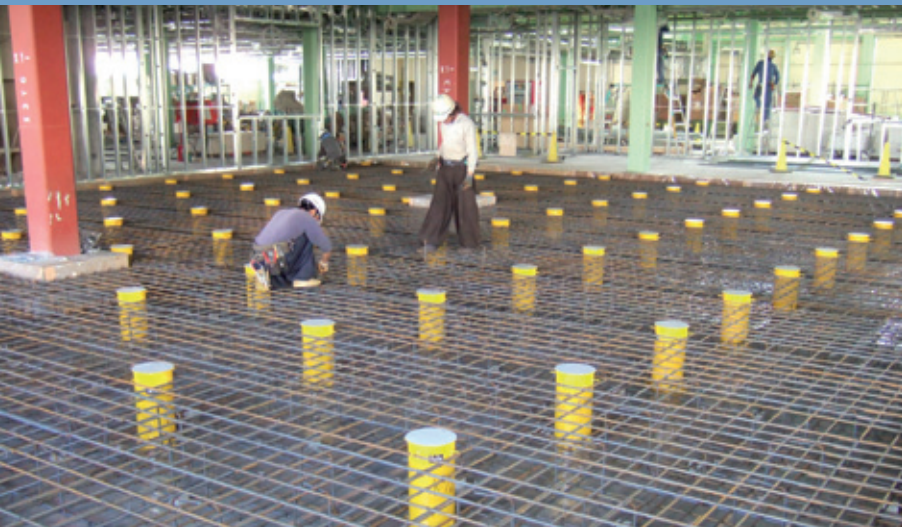
Constructing a floating floor
