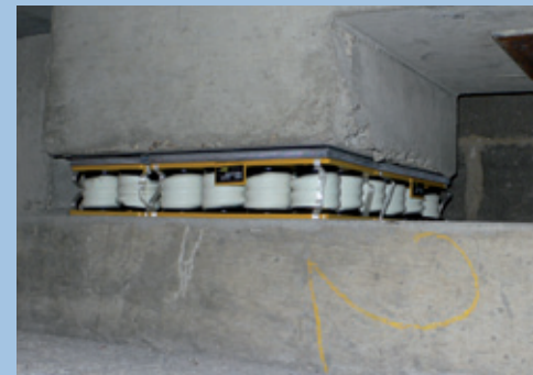
Spring support of an anechoic chamber
