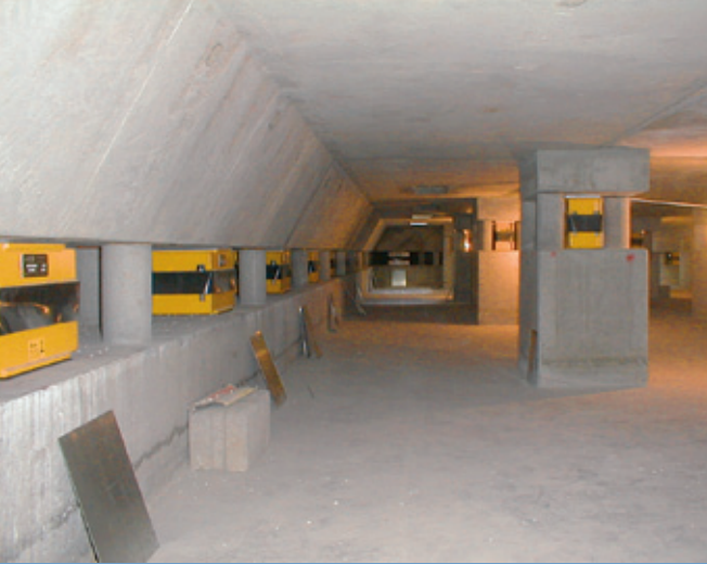
Spring support of a TV production room
