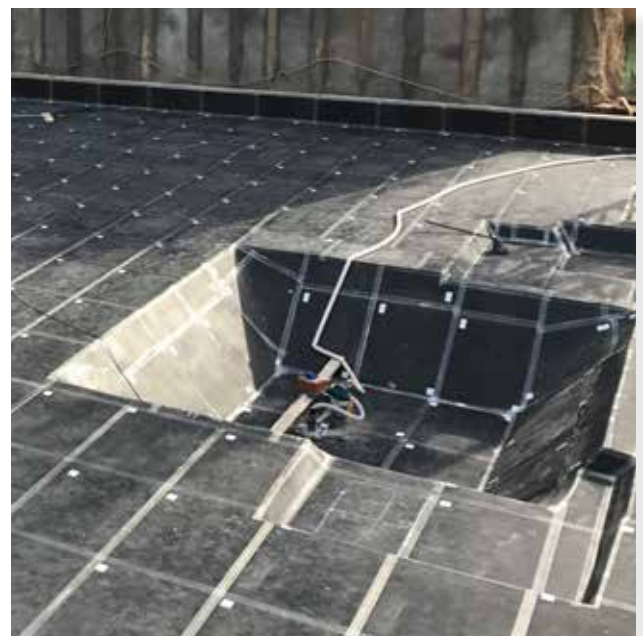
Full-surface support NOVODAMP®, Beijing, China
