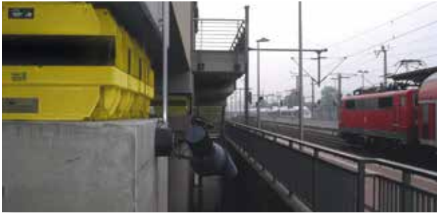
Spring supported cinema building close to a railway station, Siegburg, Germany
