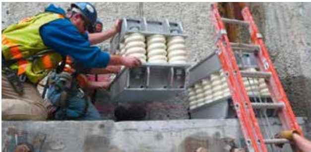
Positioning of prestressed spring elements, Boston, USA
