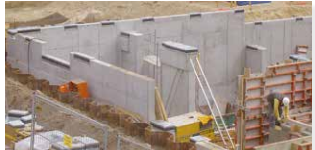
Spring elements to support a townhouse close to a metro line, Berlin, Germany
